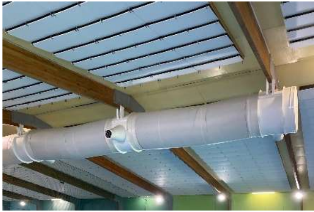
a. Bespoke louvre panel design allowing air flow in the roof cavity
